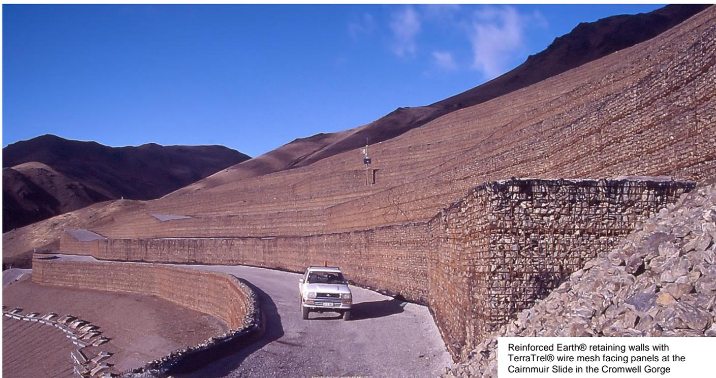
Reinforced Earth® retaining walls with TerraTrel® wire mesh facing panels at the Cairnmuir Slide in the Cromwell Gorge
