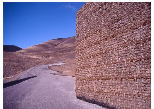
Main picture and above: Reinforced Earth® retaining walls, with TerraTrel® wire mesh facing panels, at the Cairnmuir Slide. Cromwell Gorge - Central Otago,
