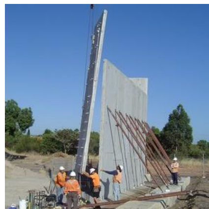
Main: TerraTilt® at Kwinana Freeway Interchange. Top: TerraTilt® at Karel Avenue Interchange. Center: TerraTilt® at South Street Interchange. Above: Installation of TerraTilt® panels.
