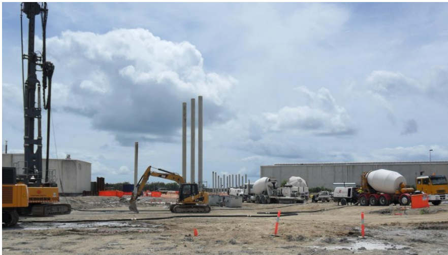
Left: Construction of the Controlled Modulus Column (CMC). Above: Reinforced Earth™ straps are being placed during the construction of the TerraPlus® Reinforced Earth™ walls.
