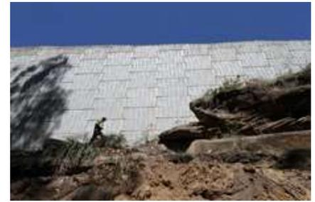
**Left:** A completed section of the TerraPlus® panel wall with a vertical rib finish
