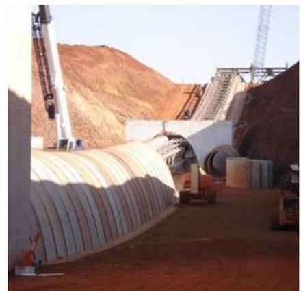
Installation of TechSpan® reclaim tunnel with a variable vertical alignment of up to 10% grade adding significantly to the design complexity and requiring wider arch units to ensure longitudinal arch stability.
