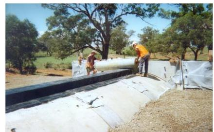
Main Picture: Saturday 16h00: TechSpan® Arch Tunnel erection completed.
