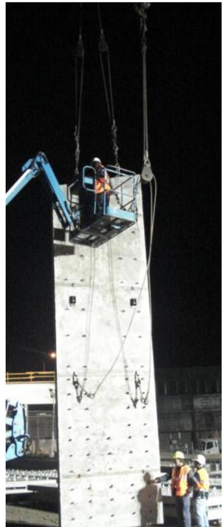
TerraTilt® full height panels are installed for the first time on Australia's east coast, quickly creating a safe working environment adjacent to a heavily trafficked suburban railway line at Gateway South.
