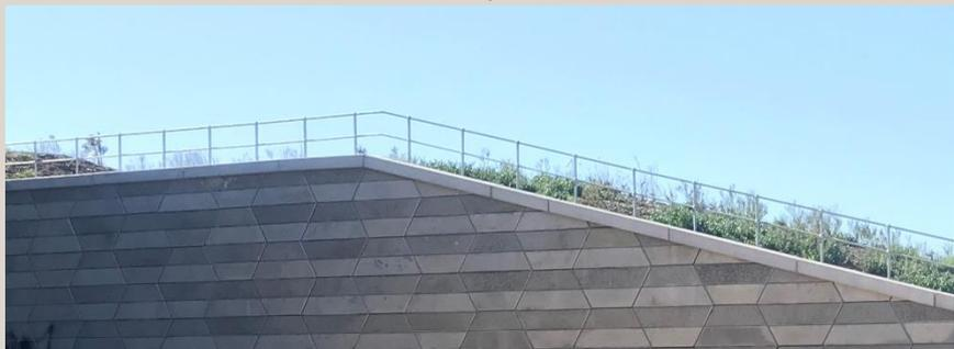
**Above:** Reinforced Earth® Abutment walls with precast capping units
