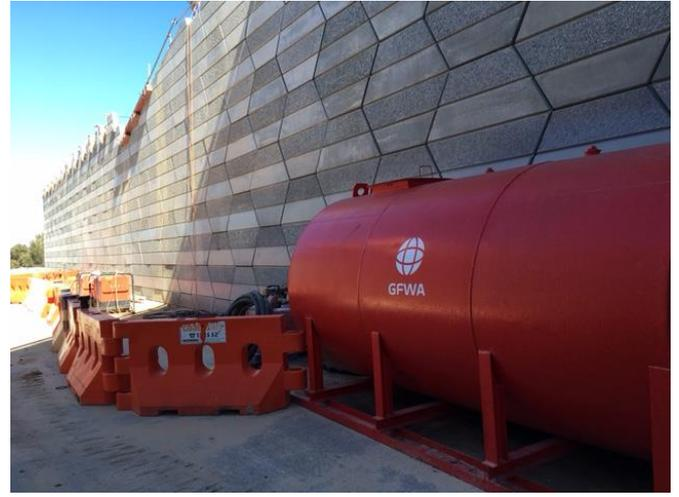
**Above on the left:** Reinforced Earth® TerraTilt® walls with hexagonal pattern
