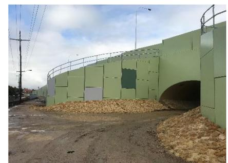
**Main:** Completed Nicholson Road bridge with Reinforced Earth® abutments and wingwalls – courtesy of MRWA website
