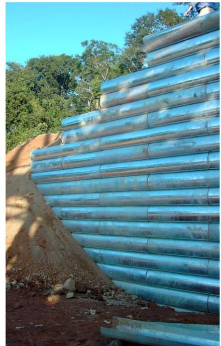
Main Picture: Sepon Copper – View of backfill, reinforcing straps, gravel drain behind structure, front face and panels ready for installation.
