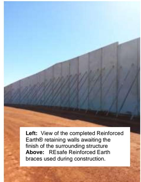
**Left:** View of the completed Reinforced Earth® retaining walls awaiting the finish of the surrounding structure
