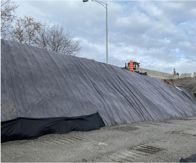
Figure 8. Installation of the DRAINTUBE behind MSE walls
