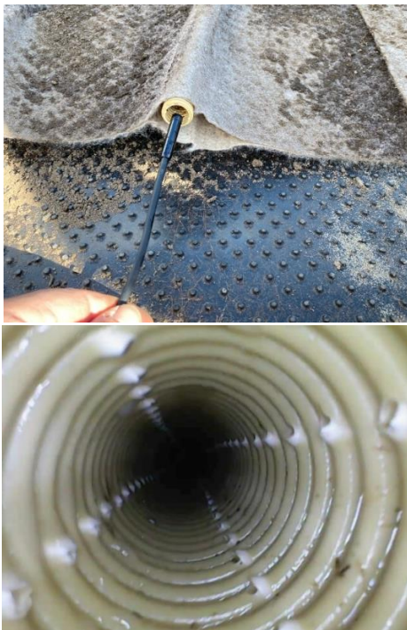
Figure 9. Example of monitoring in pipes after 12 years. Canada.
